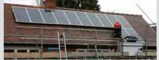
We installed solar panels which generate 3111 kwh per annum and earns us £1240 through the government Feed in and Export Tariffs. This reduces our CO2 emissions by 2.2 tonnes
