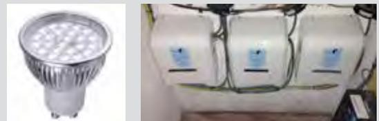
LED lights have reduced our lighting energy consumption by 75% saving £1,836 per annum and reduced our CO2 emissions by 8.81tonnes. 2 years after installation not one bulb has failed. Our new Voltage Optimization units reduce the 240 volts coming in to 220 volts as all modern electrical appliances work on 220 volts. This will save approximately 13% energy usage and extend the life of all our electrical equipment.
